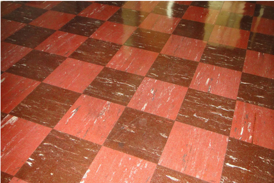
9" x 9" Asbestos Tile
